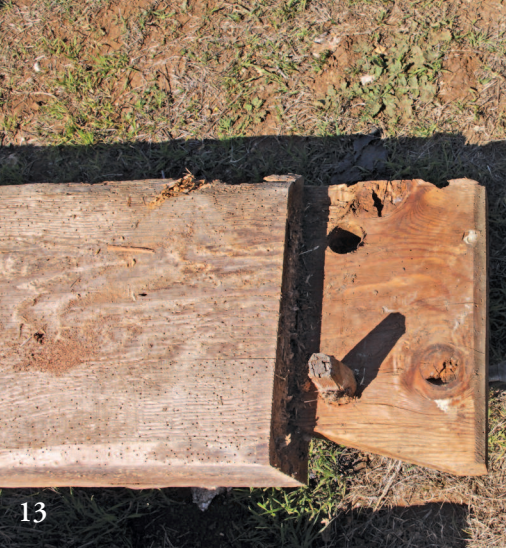
13, 14 Half-dovetail tenons at tie beam ends were wedged down onto their sloped seats in wall posts, and pinned for good measure. Wedge, not shown, fitted mortise above housing.
