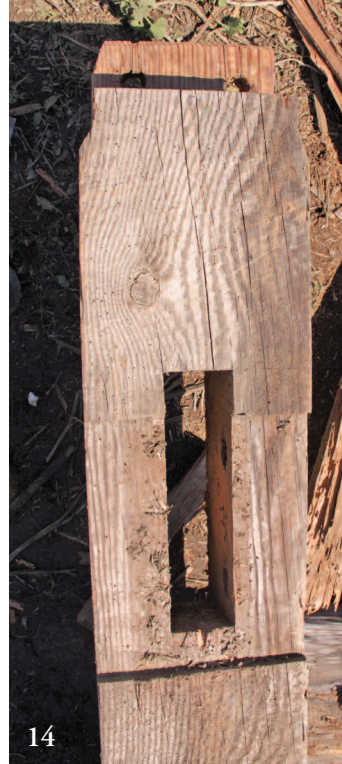
13, 14 Half-dovetail tenons at tie beam ends were wedged down onto their sloped seats in wall posts, and pinned for good measure. Wedge, not shown, fitted mortise above housing.
